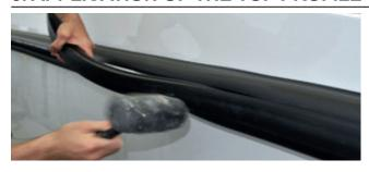
Apply the closing profile by pressing with a rubber hammer.
