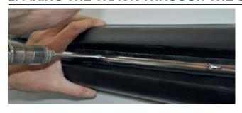
Drill holes in the boat using the same holes of the bars as a guide.
